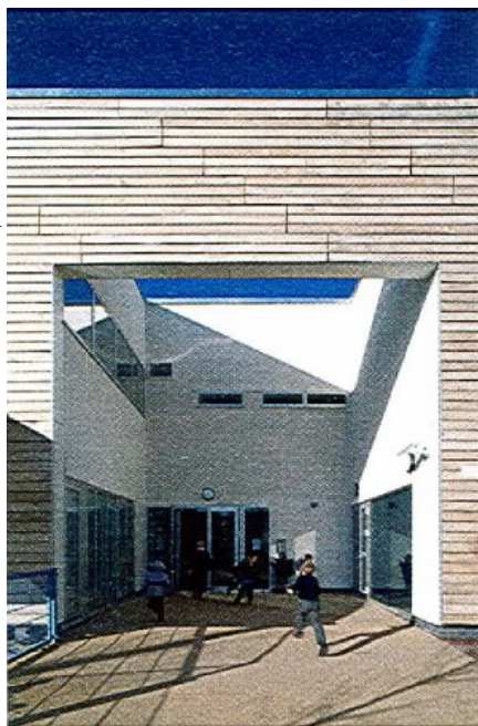
Right/above Strategically placed rooflights allow daylight to flood into the centre of the building, minimizing the need for artificial lighting of deep-plan spaces.
