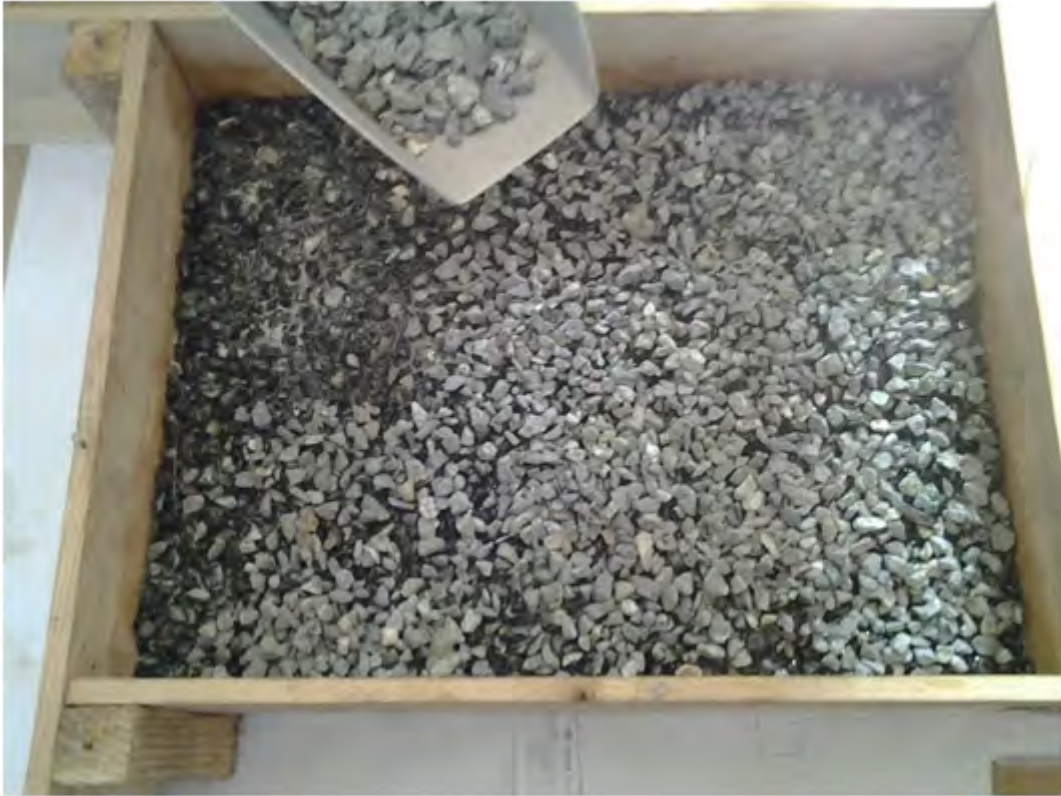
Fig. 66. Laying the 2nd aggregate layer after application of resin on the 1st layer.
