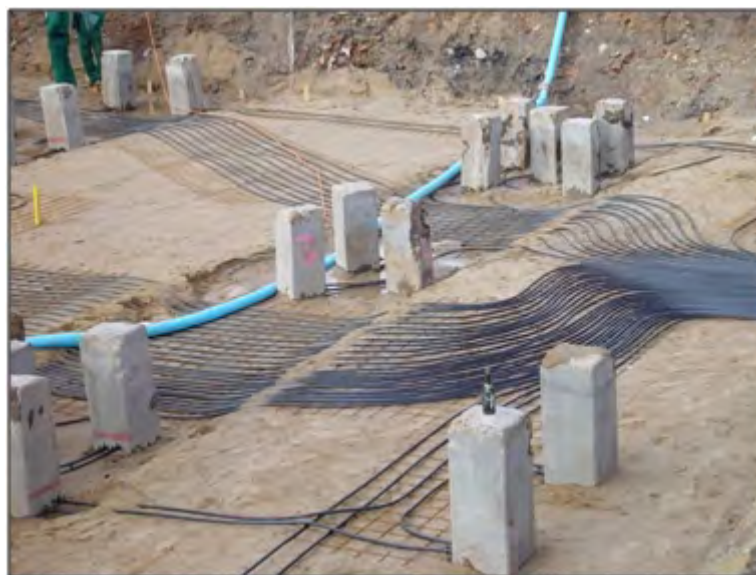
Fig. 12. precast concrete piles ("Centrum piles"), energy pile field Rostock "SILO 4+5".
