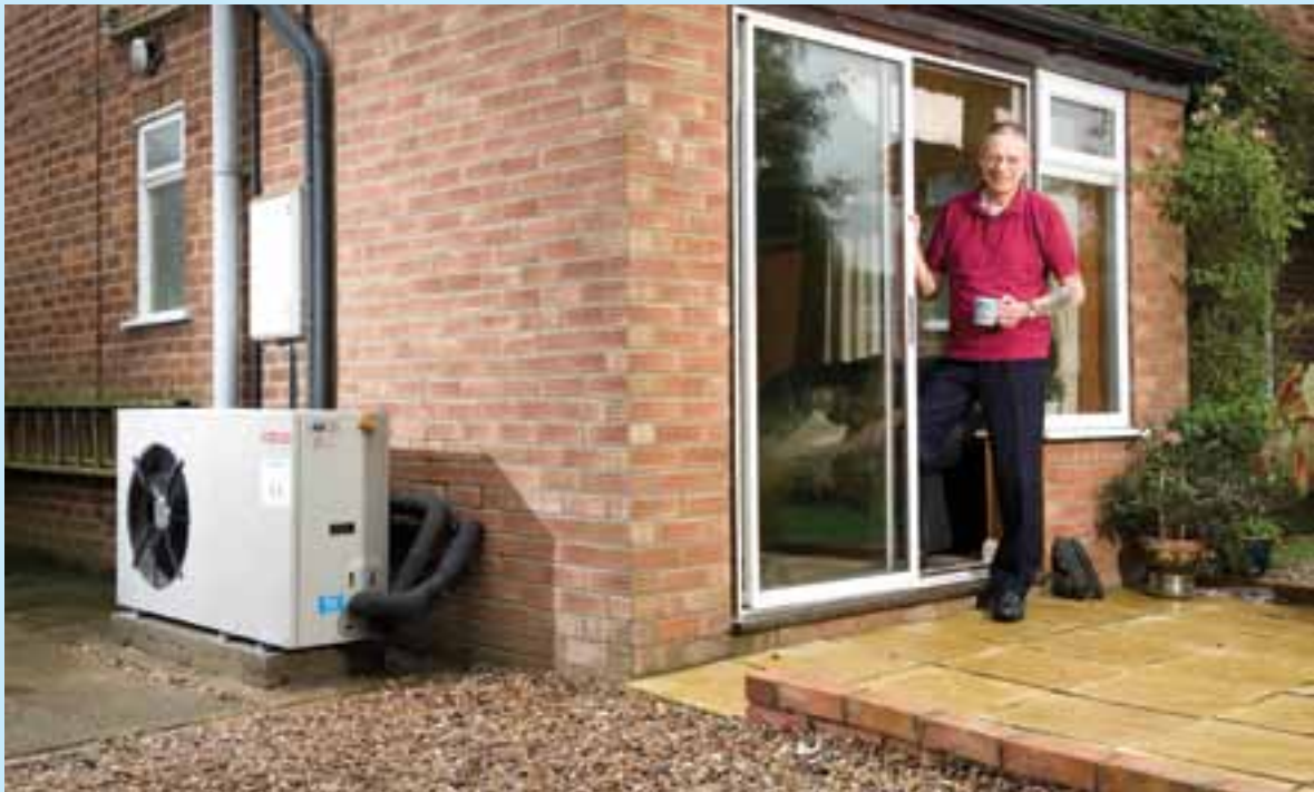
Air Source Heat Pump in situ, Ulrome
