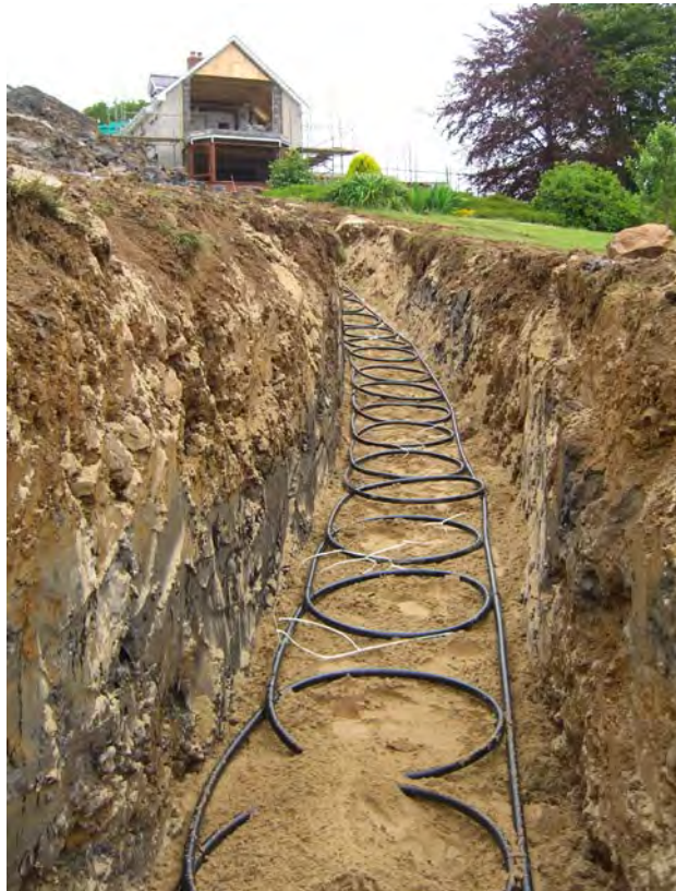
Figure 3 Trench and SLINKY™ © GeoScience
