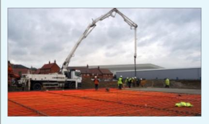
The solar heat collector pipework for the ICAX Interseasonal Heat Transfer system is shown above being installed before the playground is laid. In addition to this system, the wind turbine, solar panels and the TermoDeck building 'mass' ventilation system, the new school features...
